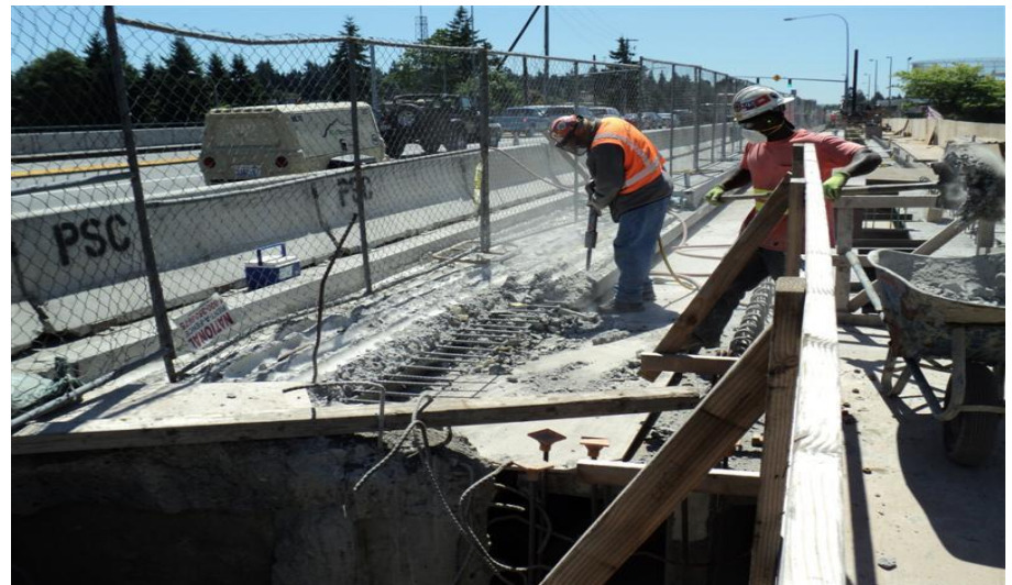
SR 99 Bridge Sidewalk and Guardrail Demolition
