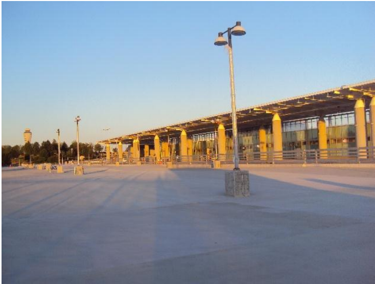
RCF Employee Parking Light Poles and Traffic Coating
